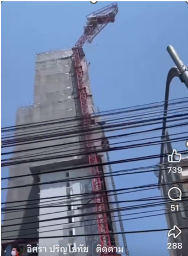
Figure 3. A Construction Tower Crane Toppling in Bangkok
