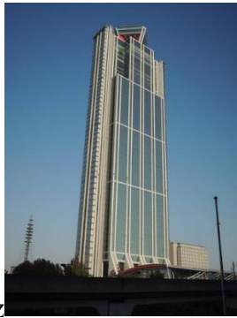
Figure 3. Sakishima Building, Osaka http://www.tanikenchiku.com/250.htm
