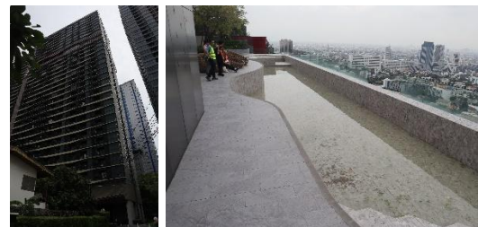
Figure 2. Example of investigated buildings and its rooftop pool.
